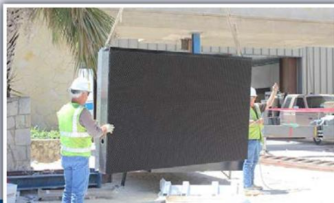
Workers ensure a module is secure prior to its being hoisted by crane to the video display panel.
