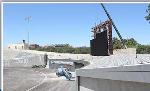
The crane then flies the module into place for the next stage of the installation process.
