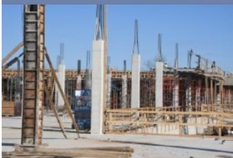
First floor concrete floor is complete, with framing on the second floor starting.
