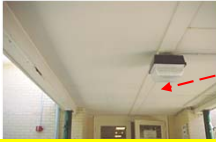
Non-Friable asbestos-containing Transite® panels
