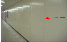
Non-Friable asbestos-containing Transite® panels
