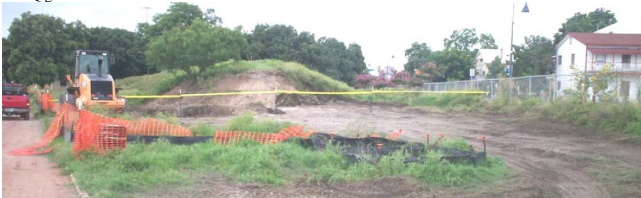
The picture above shows the environmental contractor removing the “berm” soil while the picture below shows the foundation remnants from the former high school.
