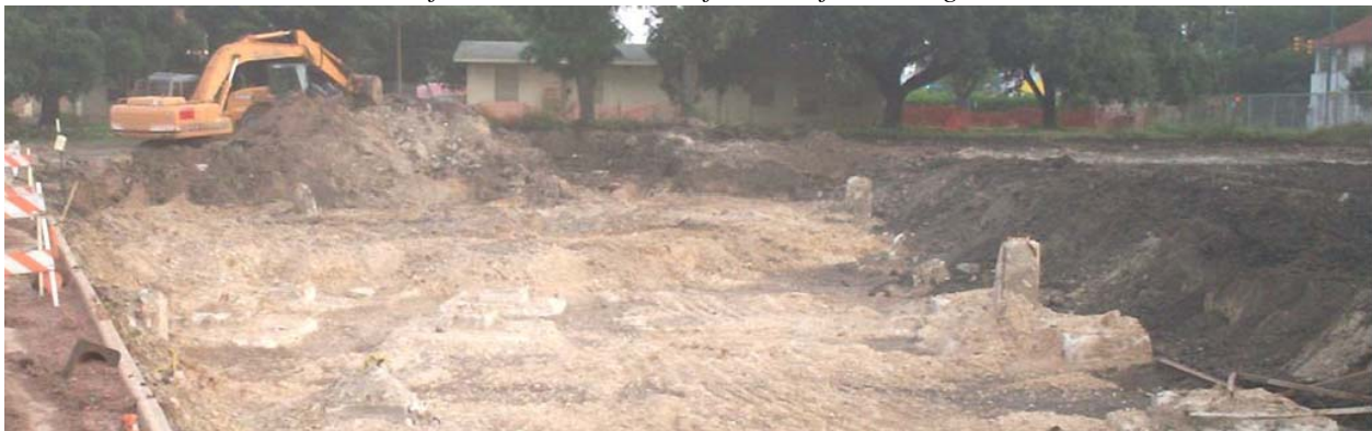
The picture above shows the environmental contractor removing the “berm” soil while the picture below shows the foundation remnants from the former high school.
