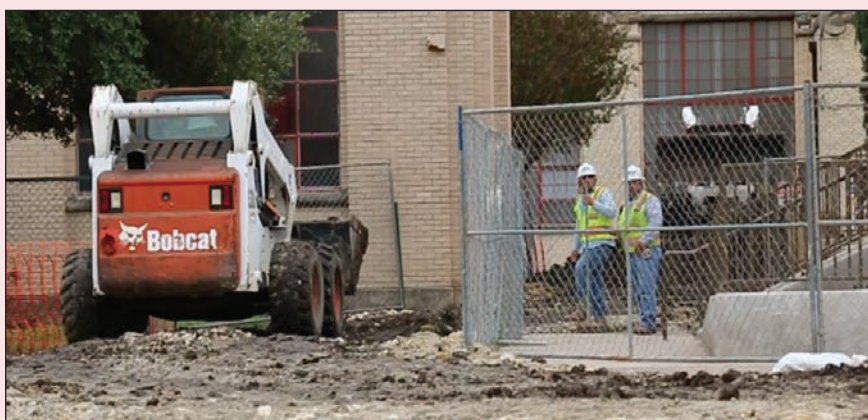
Jefferson High School construction includes renovation to the main gym, repair of the cafeteria, science corridor remodel, and interior renovations to the 1930s building including preservation of theatre and library, as well as renovation of the kitchen and dining areas.
